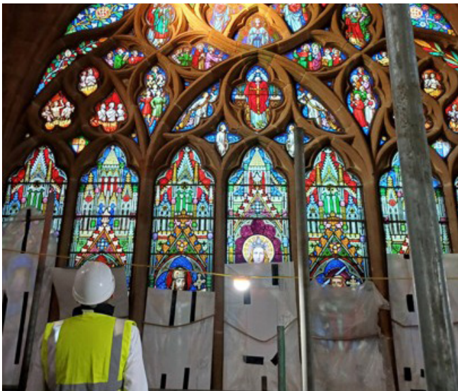
Salford Cathedral incorporates ground source heat pumps, insulation, underfloor heating, and secondary glazing. (by Purcell)
