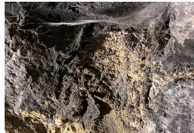
Stonework spalling
