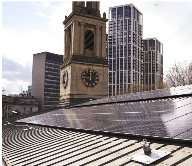
Solar panel installation at grade II* listed St John's Waterloo (Diocese of Southwark). The crypt now has electric infra-red panel heating, LED lighting, and electric kitchen appliances.
