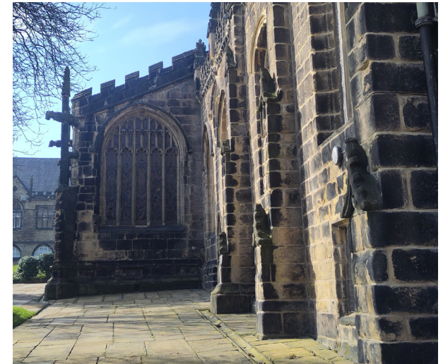
South elevation of the Minster looking west.
