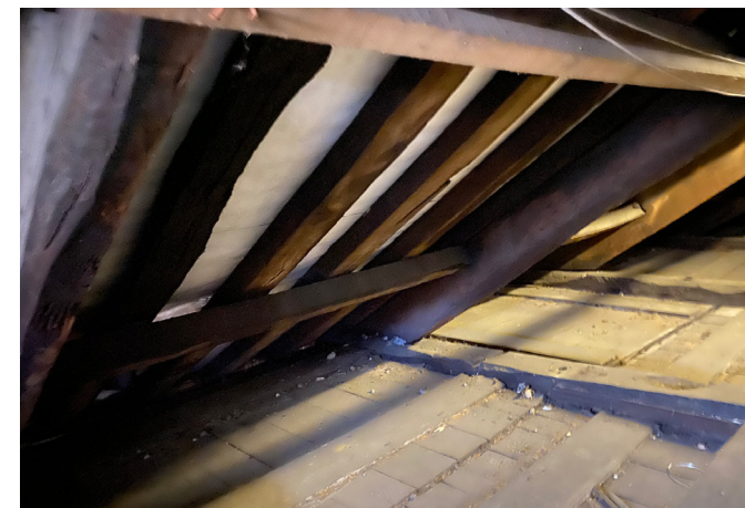
Nave roof attics
