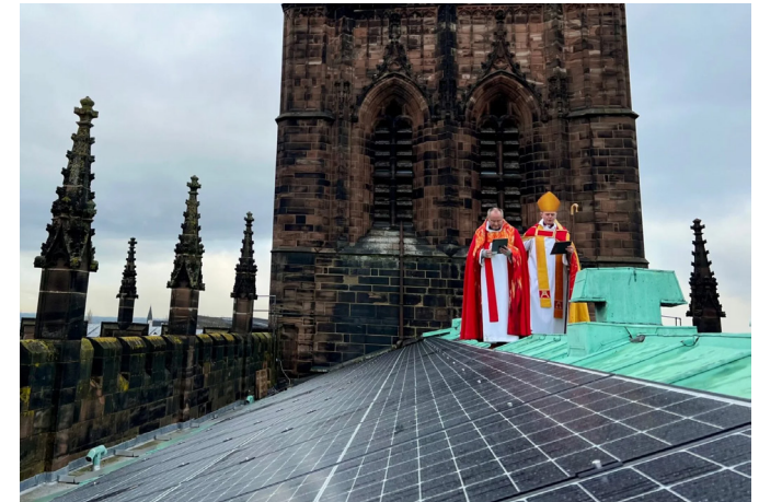
206 solar panels at Chester Cathedral generate 22-25% of the total energy consumption of the building.
