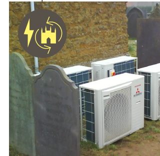
Replacement of gas boilers
