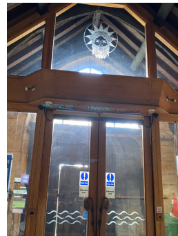
● Vestibule in good condition
