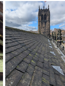
● Damaged and failing membrane
