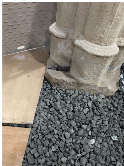
Insulation and underfloor heating being laid in Salford Cathedral
