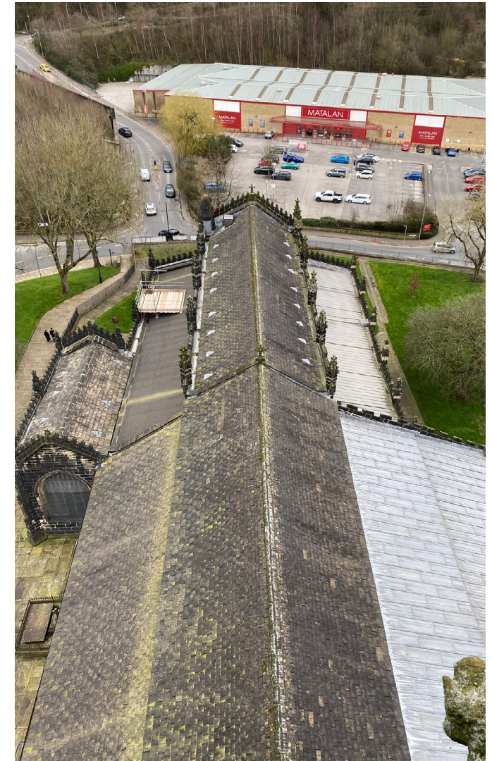
Photo of roof from tower.
